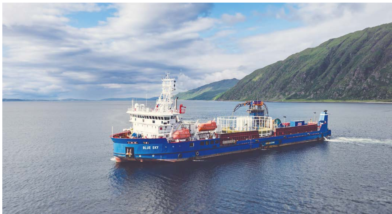
Cable laying in the Ardnamurchan Peninsula is part of the expansion of SSEN Distribution's network that will increase earnings over the long term
