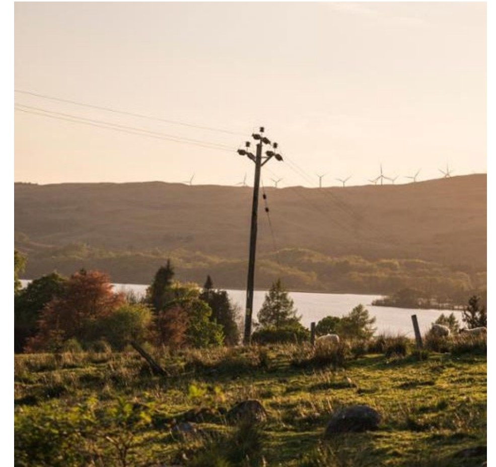
SSEN Distribution Overhead Line
