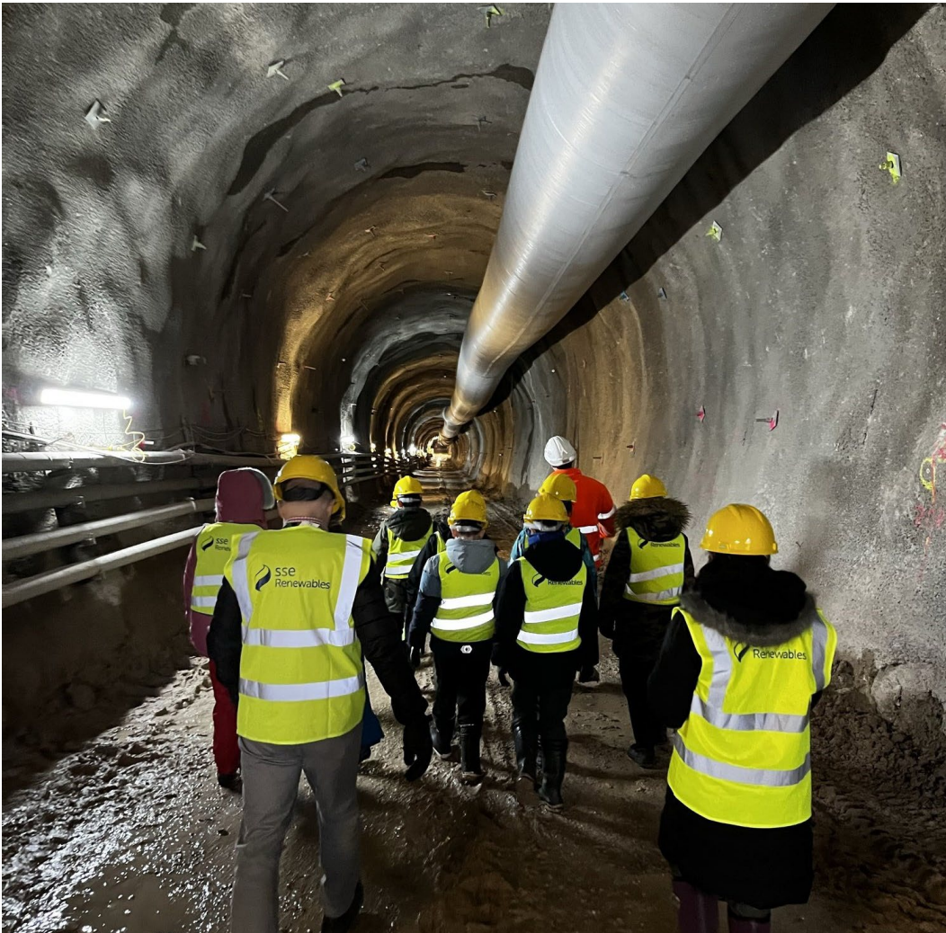
Pupils from Invergarry Primary School visiting the Coire Glas exploratory tunnel
