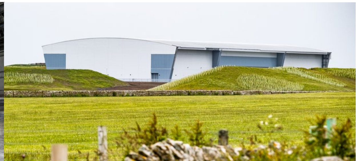
Caithness-Moray-Shetland HVDC switching station at Noss Head
